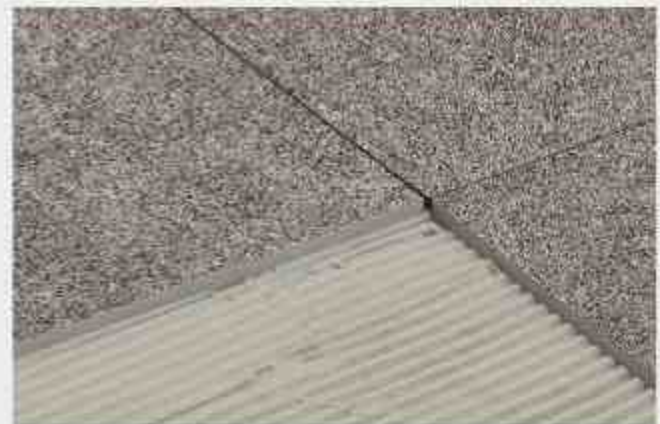
Laying with Adhesive
