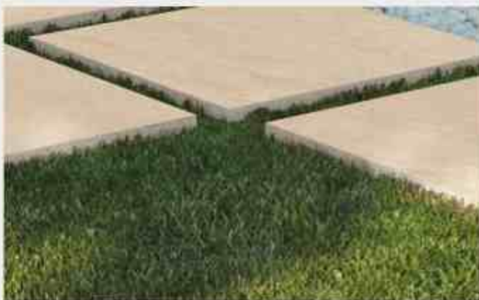
Dry Laying on Grass
