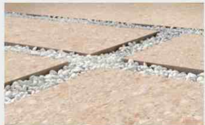
Laying on Gravel
